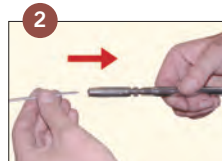
Insert cable into fitting
