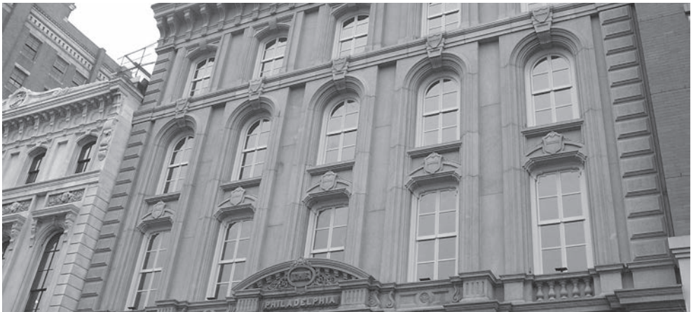
THE PHILADELPHIA BANK BUILDING – Philadelphia, PA
